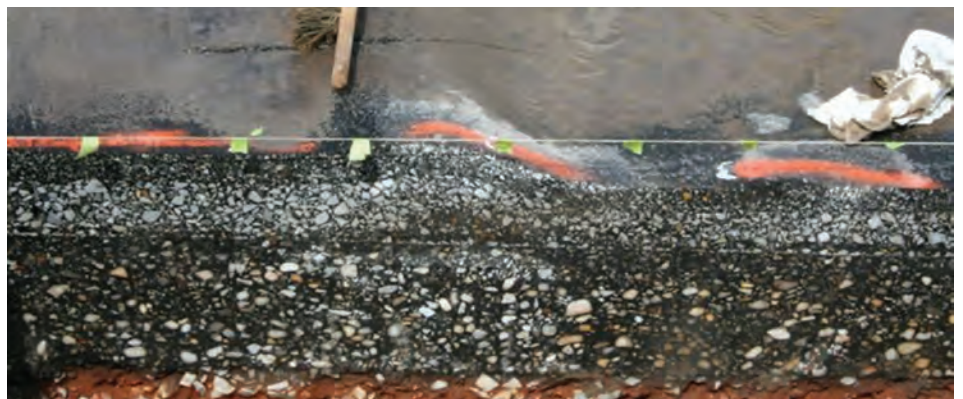
Figure 1. Rutting Observed in Binder SMA During Forensic Trenching
