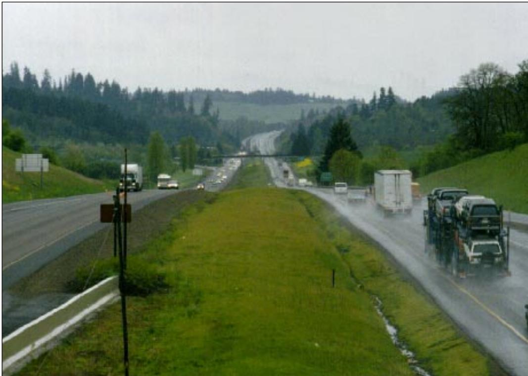
Figure 1. Interstate 5 in Oregon. Note the absence of splash and spray on southbound lanes (left) with OGFC compared to northbound lanes (right) with dense-graded HMA.
