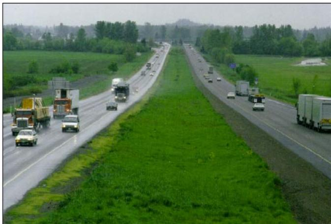
*Figure 2.* Interstate 5 in Oregon. Note the absence of glare from headlights during wet conditions on southbound lanes (right) with OGFC compared to northbound lanes (left) with dense-graded HMA.
