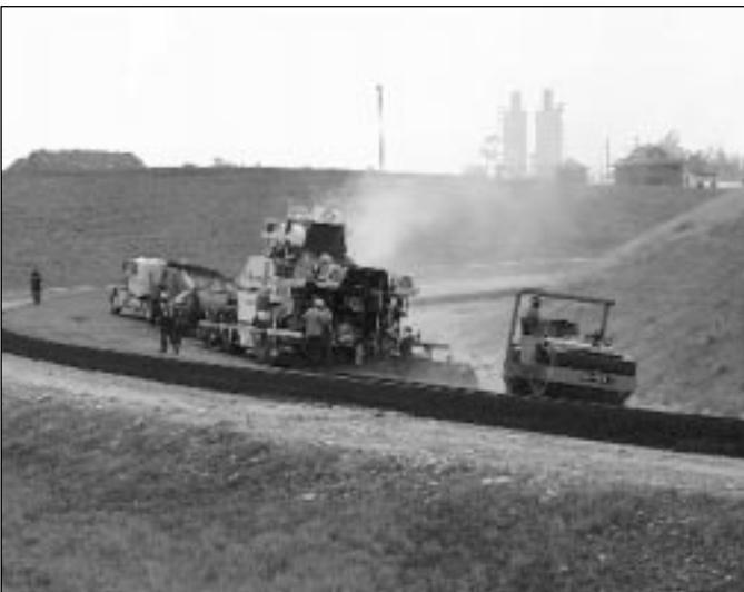
*NCAT Test Track — HMA Paving train constructing the base course*
