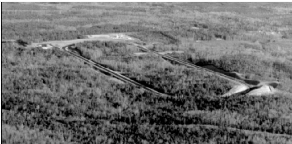
*Aerial view of the 1.7-mile, oval NCAT Test Track after HMA base course construction was completed.*
