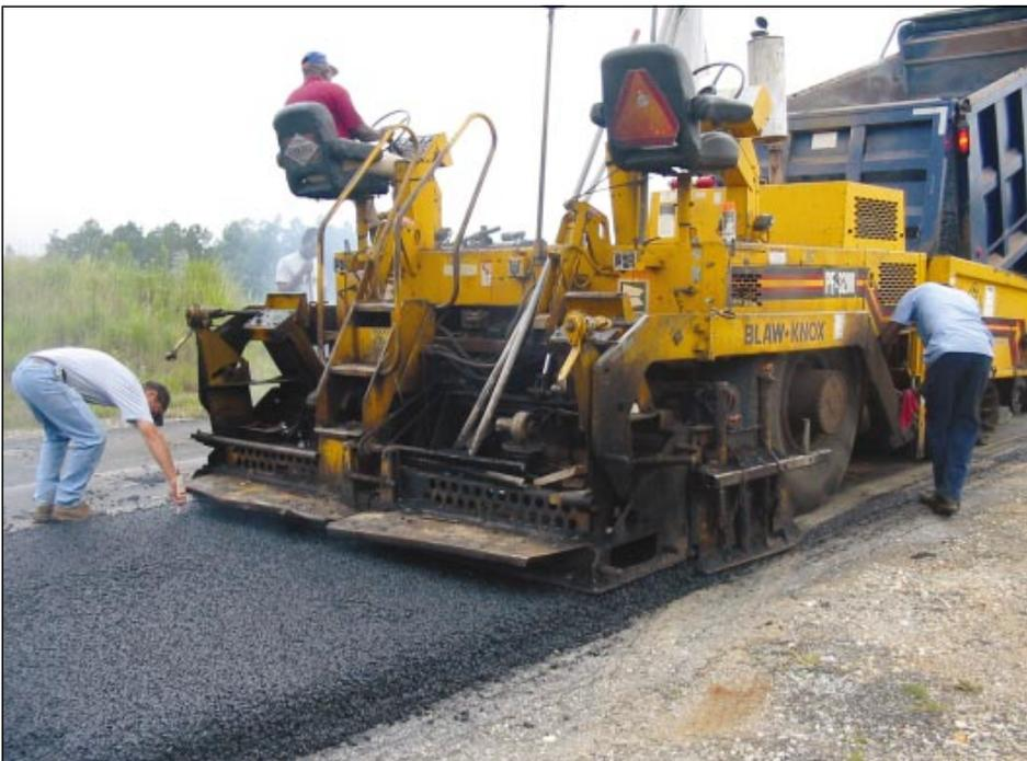
Placement of hot mix asphalt with different lift thicknesses for NCHRP Project 9-27
