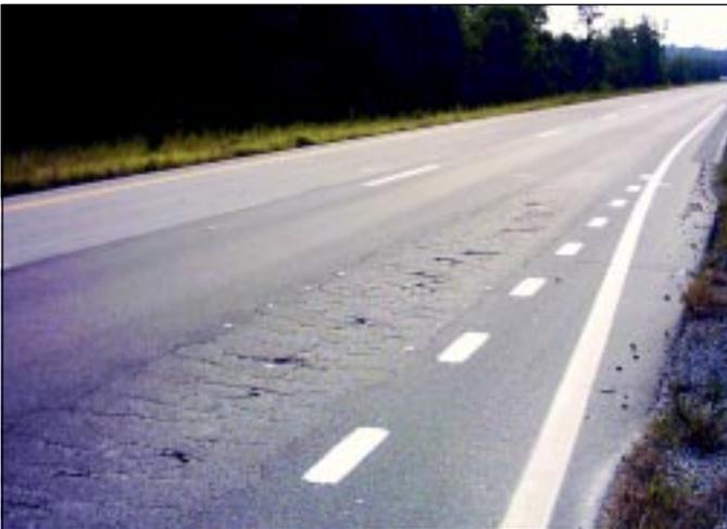
Figure A. Fatigue cracking in structural Test Section N1
