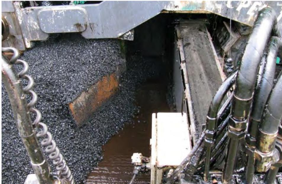
**Figure 1 Applying Thick Polymer-Modified Tack Coat Using Spray Paver**
