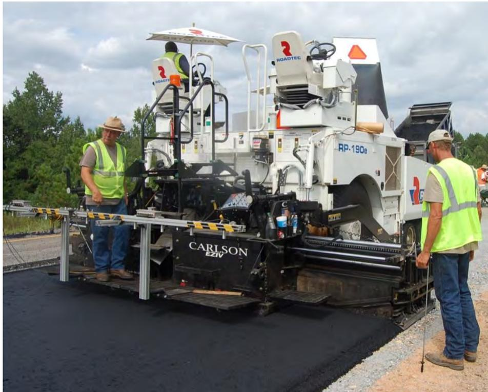
**Figure 3 Paving the Base Layer of a Test Section on the 2012 NCAT Test Track**
