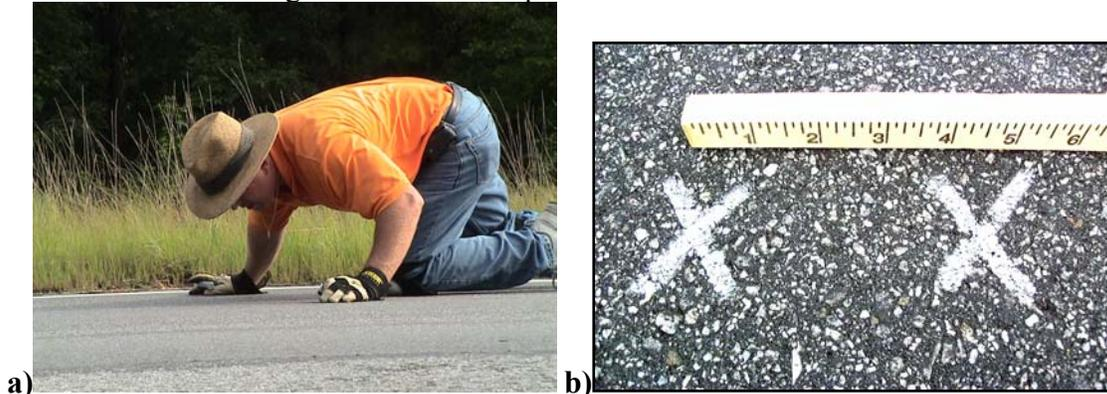
Figure 3.9 a) Pavement Inspection and b) Crack Marking.
