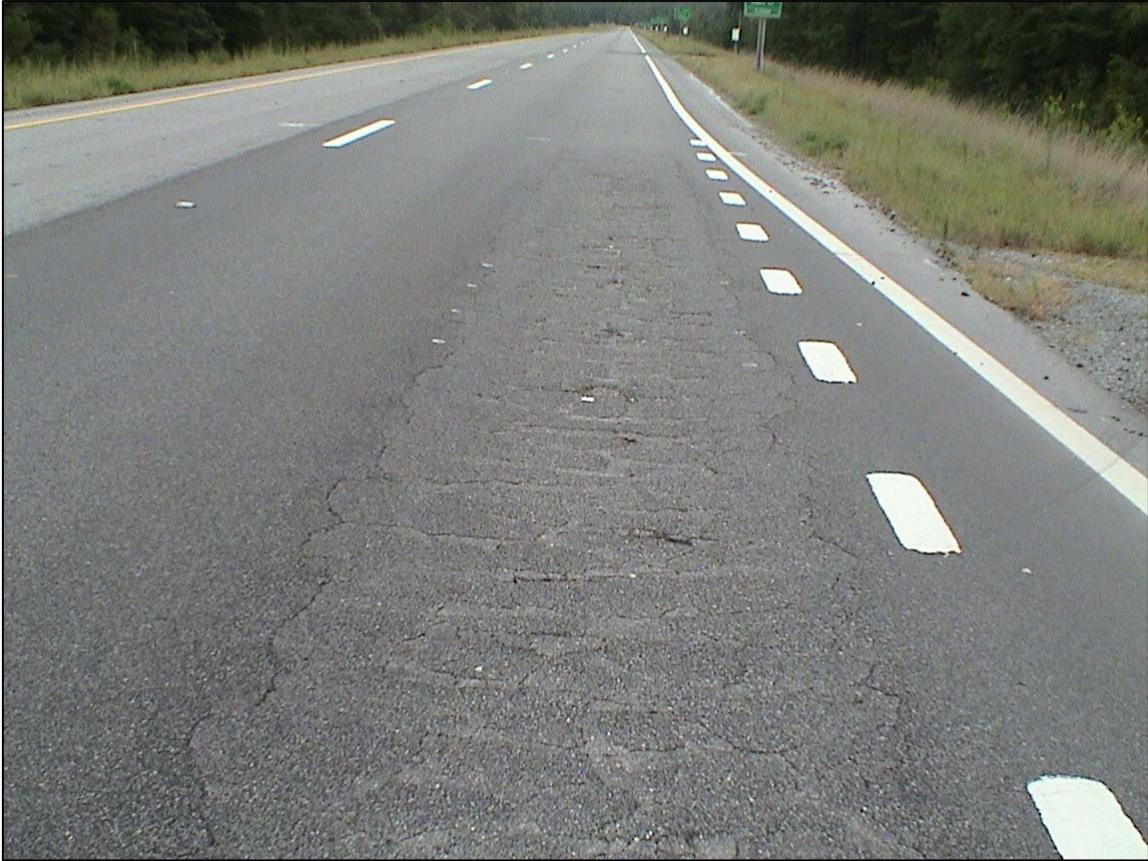
**Figure 2.3 Photograph of Fatigue Cracking.**
