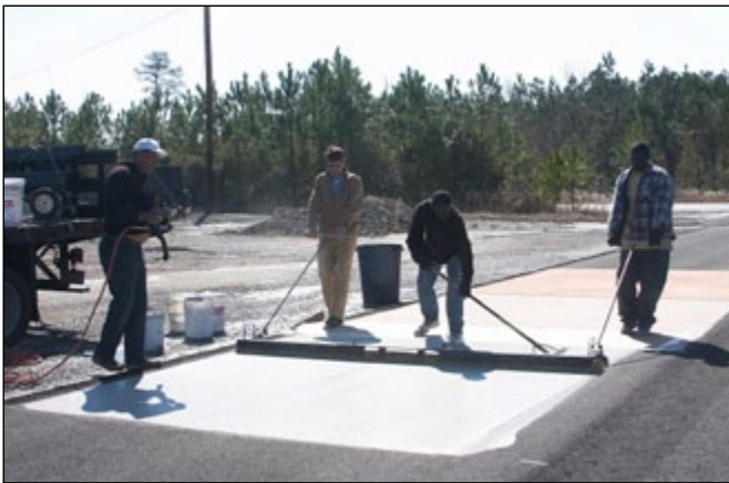
Figure 1 Installation of E-Krete® test section.
