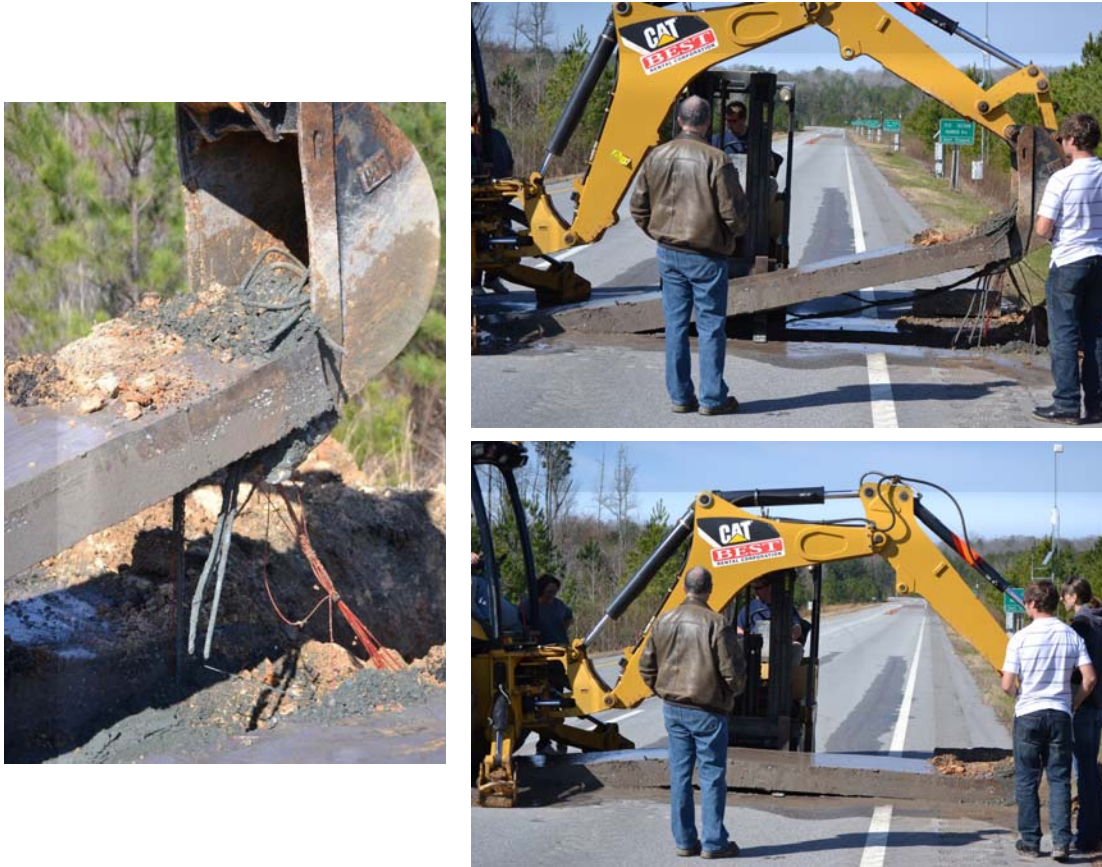
Figure 5.7 Lifting and Extracting Slab from Trench 2
