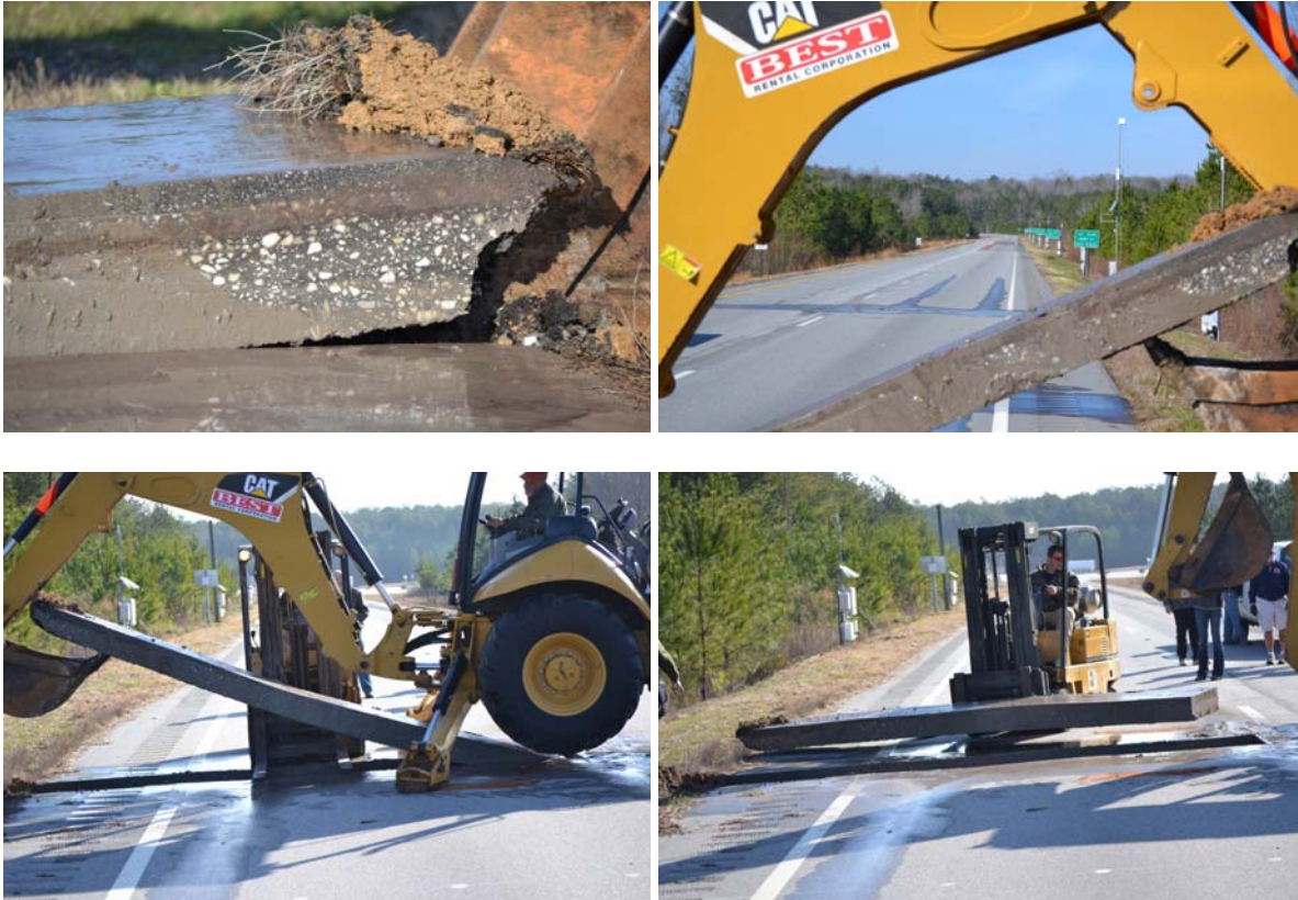
Figure 5.6 Lifting and Extracting Slab from Trench 1
