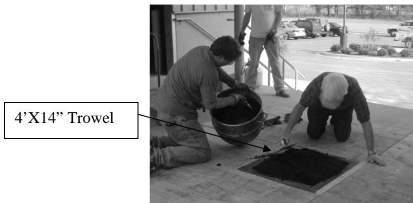
Figure 10. Distributing Mix Evenly in Mold
