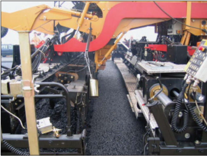
Two screeds in operation
