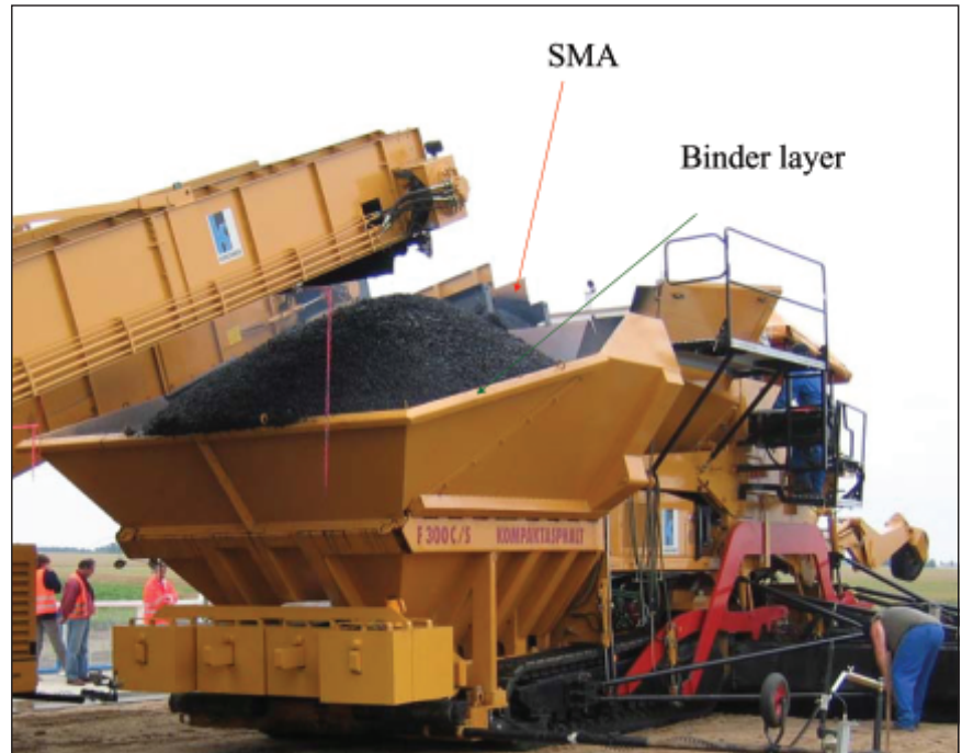
SMA and binder layer mix being fed separately into paver hoppers
