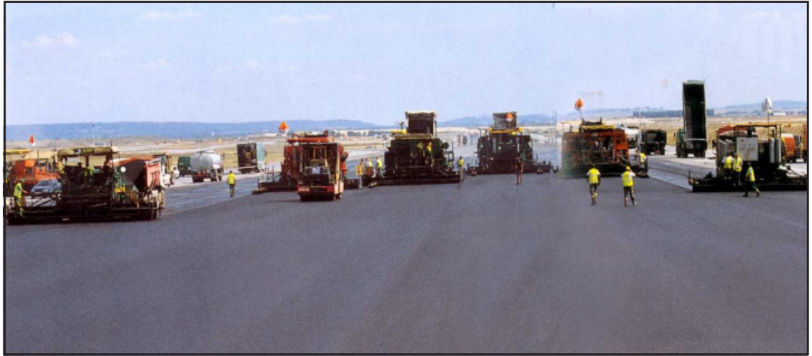
HMA paving in echelon in Chicago's Orly Airport
