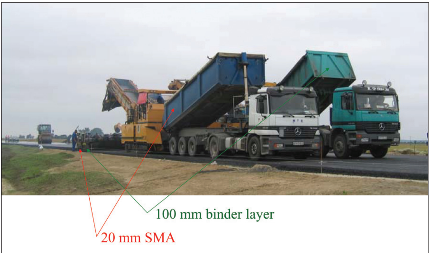
General view of the Compact-asphalt paving train
