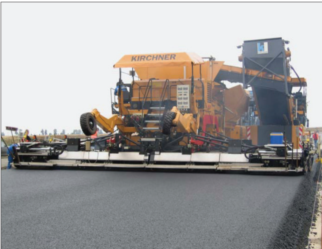
Mat behind the paver consisting of binder course and SMA
