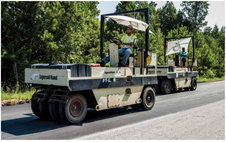
Pneumatic tire rollers are used on the NCAT Test Track to achieve proper compaction and in-place density.
