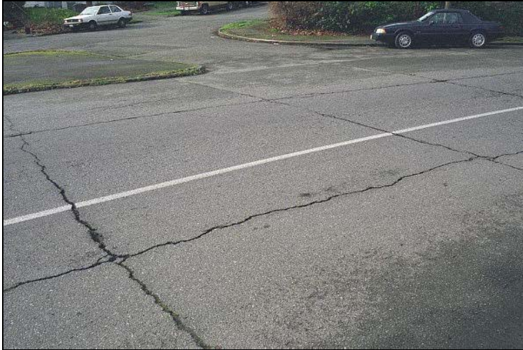
Figure 2.1 Reflective Cracking.
