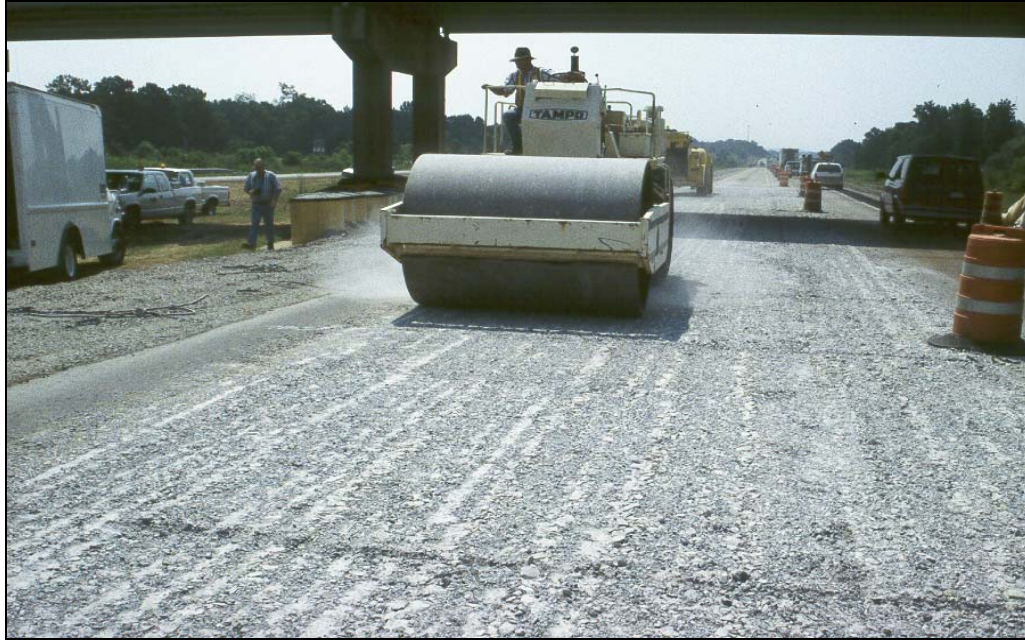
Figure 2.7 Seating the Pavement (photo by Kevin D. Hall, University of Arkansas).
