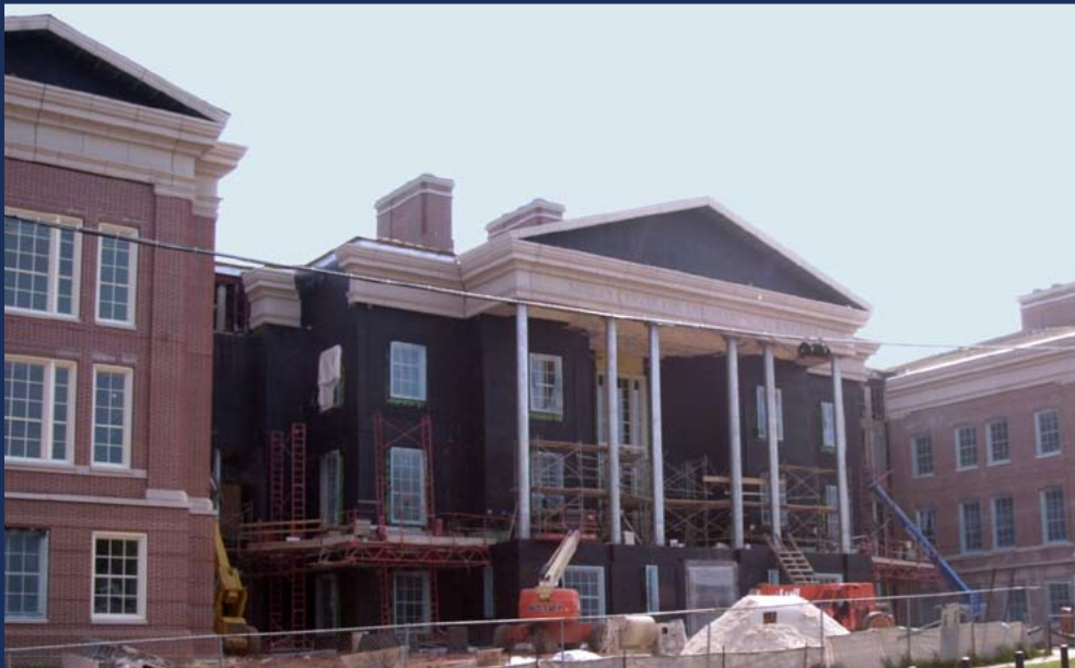
Recent construction photo of the Shelby Center
